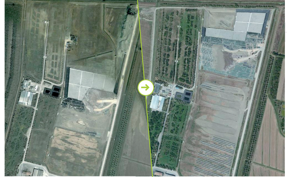
Figure 21: Aerial photographs of the dump, before installation (left) and after the completion of the first batch of 1 MW photovoltaic ground plant (right)
