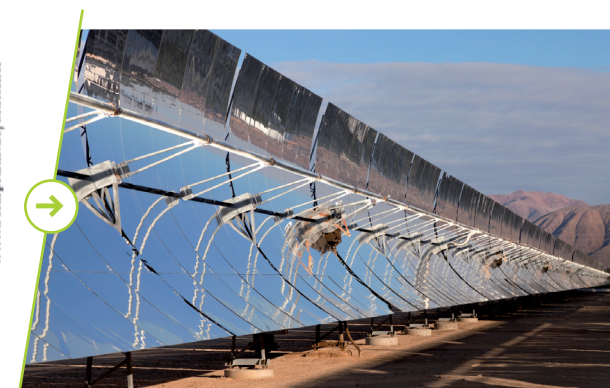
Solarlite GmbH: Parabolic trough collector
